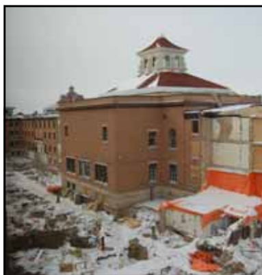
Construction has started on the New Conklin Theatre
